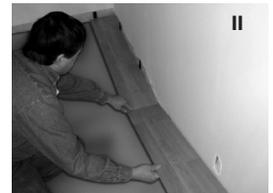
The cut piece from the first row becomes the starting piece for another row. Install the cut edge facing the wall, with the expansion wedge in place. Now angle this piece and click it into the first plank of the first row. The cut pieces should be a minimum of 8" (20cm) in length (III). Continue the second row with a full piece, placing the tongue of the long side into the groove of first row piece (IV).
