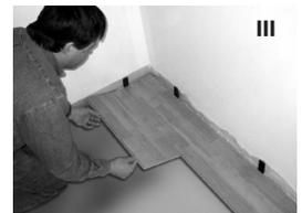
Move the end joints together until they are approximately 1/4" (6mm) apart. Click the plank lengthwise into place. For the short and long edge, use the tapping block and a number of smaller taps until the planks lock into place completely.
