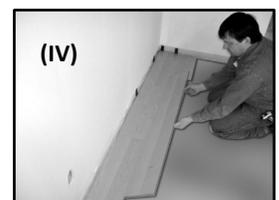
Move the end joints together until they are approximately 1/4" (6 mm) apart. Click the plank lengthwise into place. For the short edge, use the tapping block and a number of smaller taps until the planks click into place completely.
