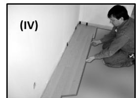
Move the end joints together until they are approximately 1/4" (6 mm) apart. Click the plank lengthwise into place. For the short edge, use the tapping block and a number of smaller taps until the planks click into place completely.
