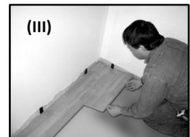
The cut piece from the first row becomes the starting piece for another row. Install the cut edge facing the wall, with the expansion wedge in place. Now angle this piece and click it into the first plank of the first row. The cut pieces should be a minimum of 8” (20 cm) in length (III). Continue the second row with a full piece, placing the tongue of the long side into the groove of first row piece (IV).
