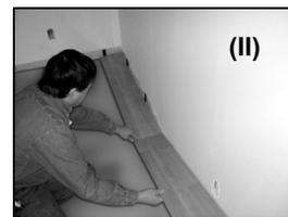
The cut piece from the first row becomes the starting piece for another row. Install the cut edge facing the wall, with the expansion wedge in place. Now angle this piece and click it into the first plank of the first row. The cut pieces should be a minimum of 15" (38 cm) in length **(III)**.
