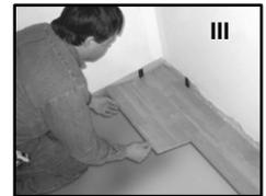
Move the end joints together until they are approximately 1/4" (6mm) apart. Click the plank lengthwise into place. For the short and long edge, if necessary, use the tapping block and a number of smaller taps until the planks lock into place completely.
